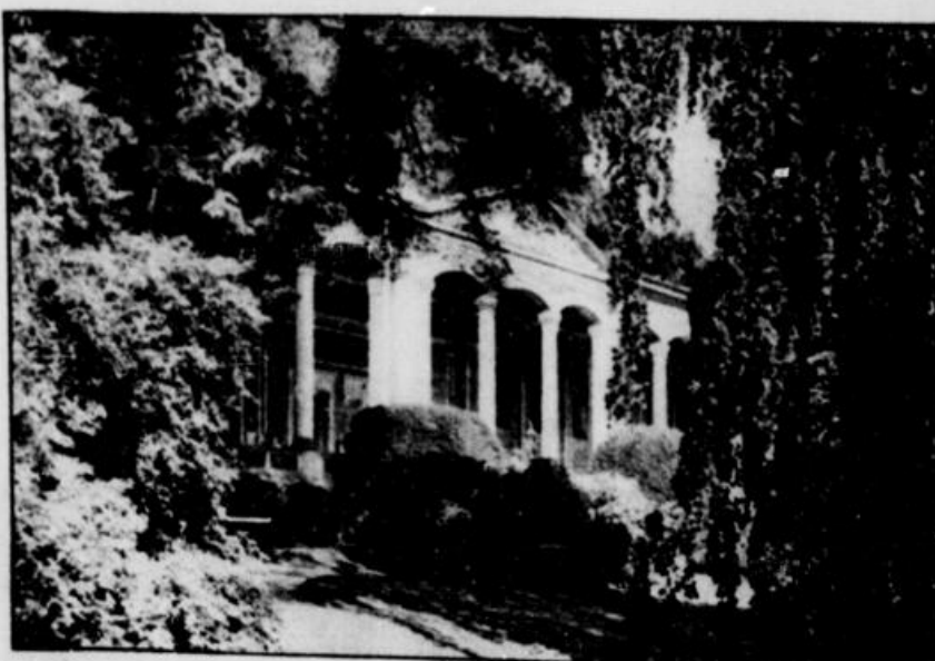
Brunnenhalle in Hohen-Hohen
